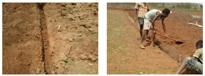
Picture S8: Trench for sheet metal and plot delineation by sheet metal
